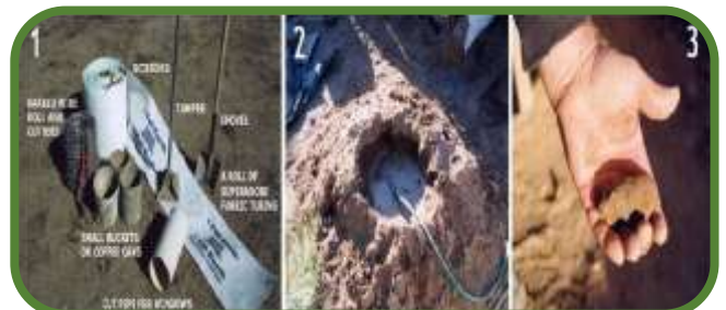
Figure 4: shows the tools used in building Earthbag houses and the method of mixing the materials that make up the filler and checking the quality of the soil before placing it in the bags
