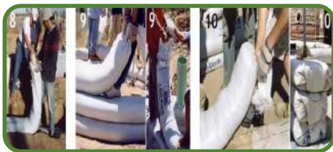
Figure 6: This picture shows how to fill and arrange the bags. Source: https://syrianchange.wordpress.com
