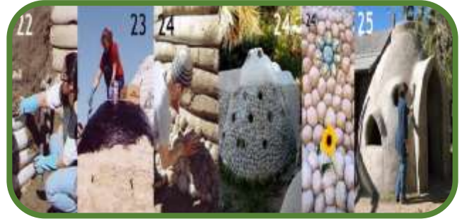
Figure 11: The pictures show a group of ways of exterior cladding for the house
