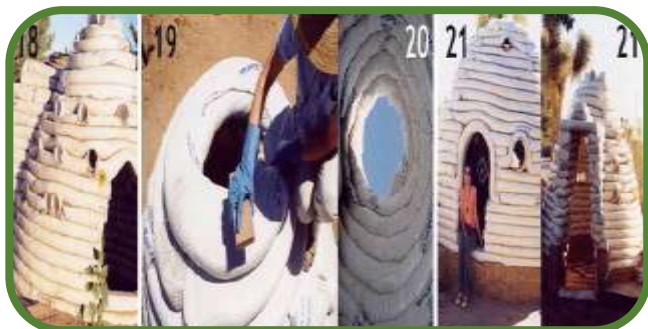
Figure 10: The picture shows the last layer of the dome building (the ceiling of the room in Earthbag houses) and the entrance to the house with the arch
