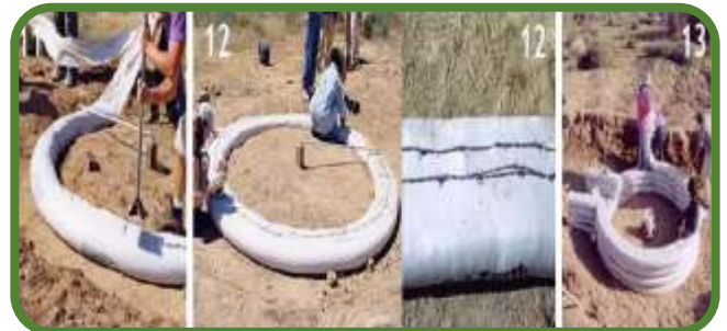
Figure 7: This group shows the process of reinforcing with wires between the layers of the bags Source: https://syrianchange.wordpress.com .
