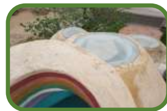
Figure 12: Skylight vents from the top of the house from the outside
